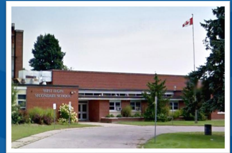
West Elgin Secondary School 139 Graham Road, West Lorne ON
